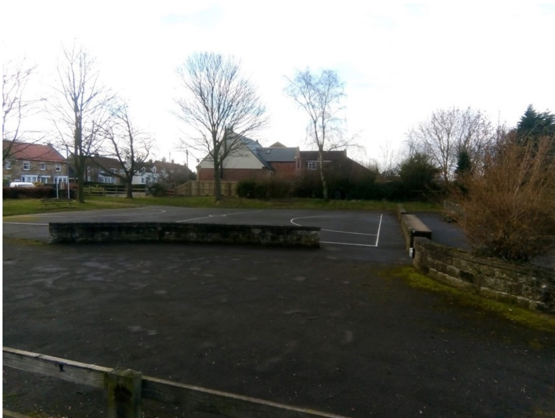
Internal view of the site showing the blank gable of the adjoining converted Chapel
