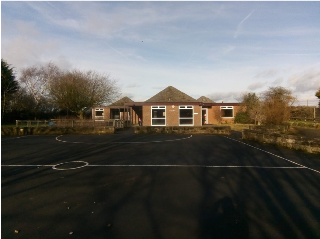
View of the existing former Ingleby Arncliffe Primary School buildings
