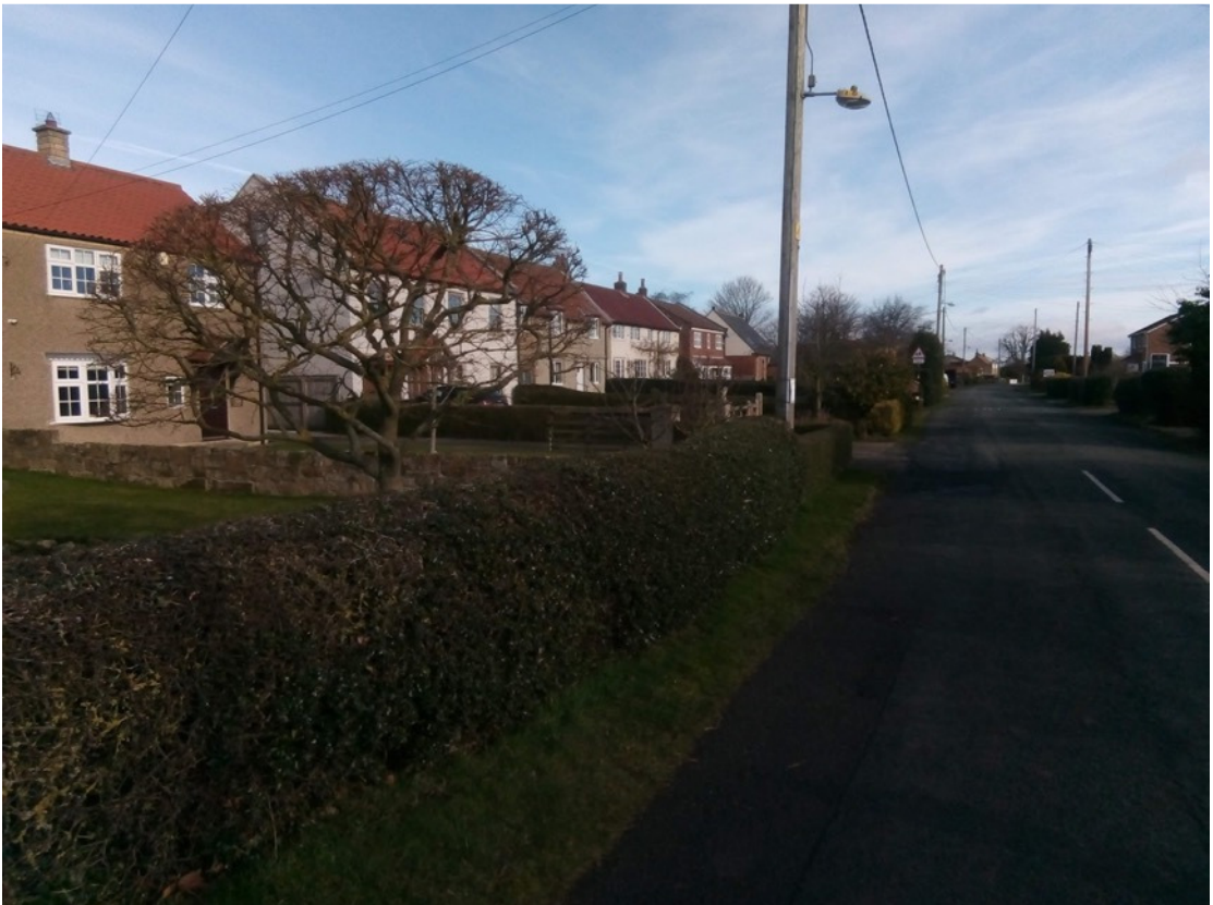
Typical street view
